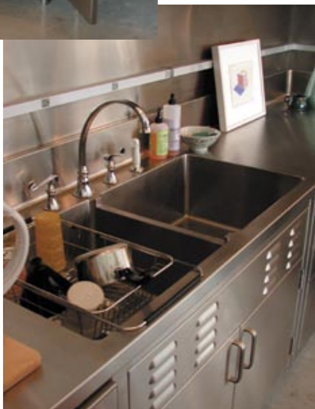
right: Counter top and sink are a single unit with louvers underneath to allow for air flow.
